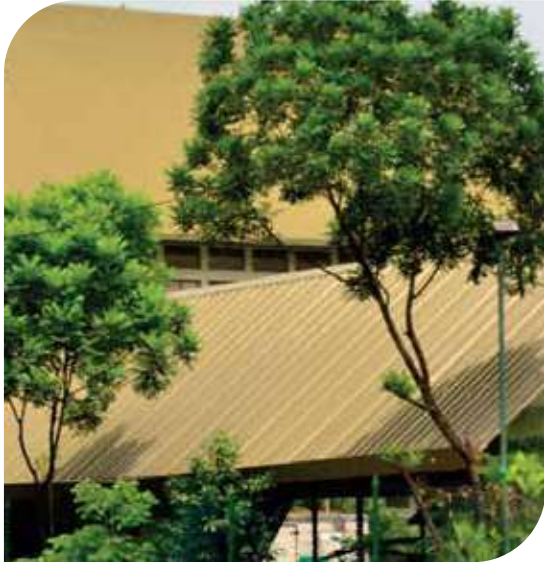
Environment Authority Buliding Supply Year - 1998
